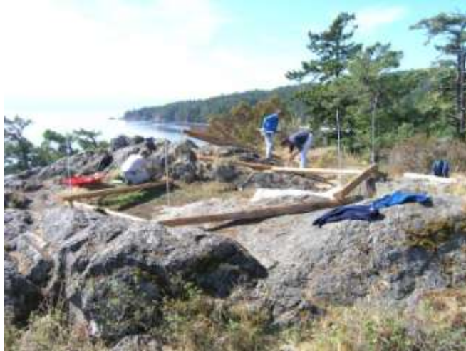
Figure 4. Crew constructing fence around vernal pool.
