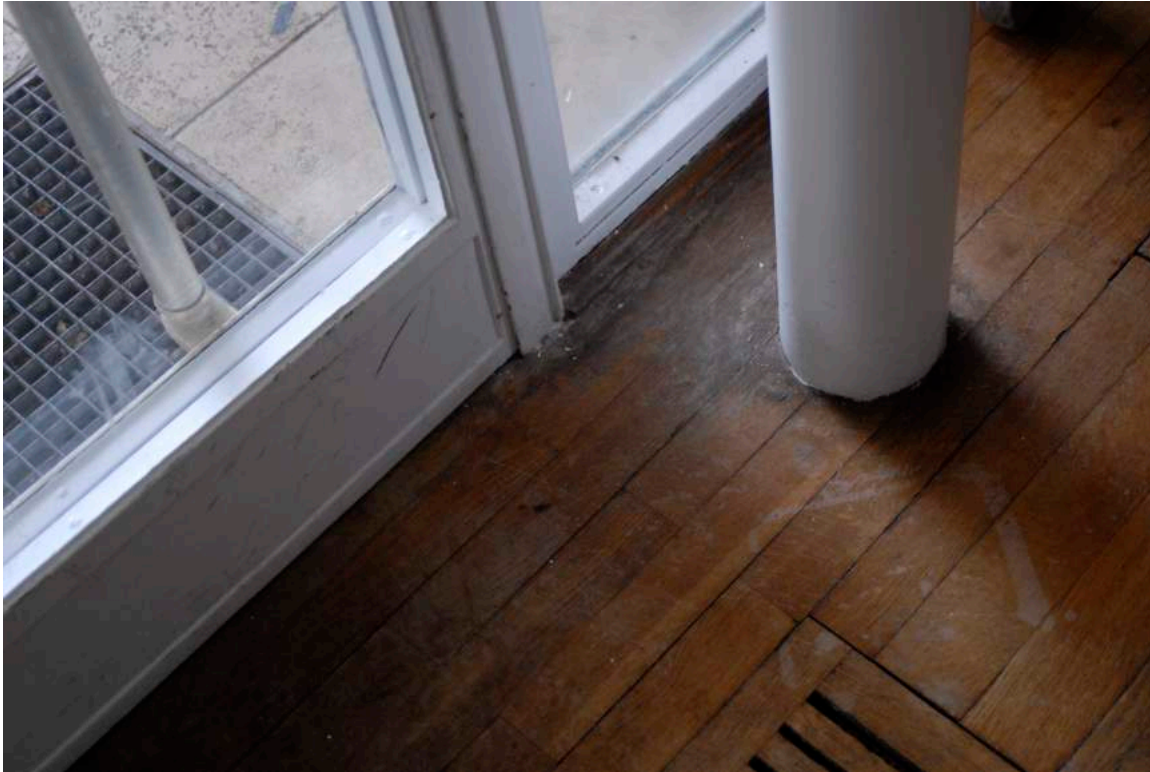
Photo of floorboards and steel framed façade. 2011. Photo by author
