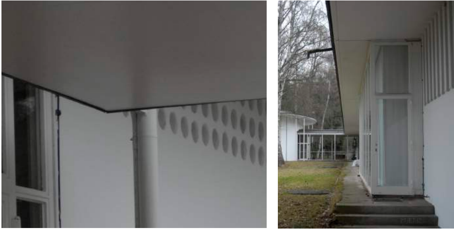
Akademie der Künste Porte-cochere and scupper details. 2011. Photos by author
