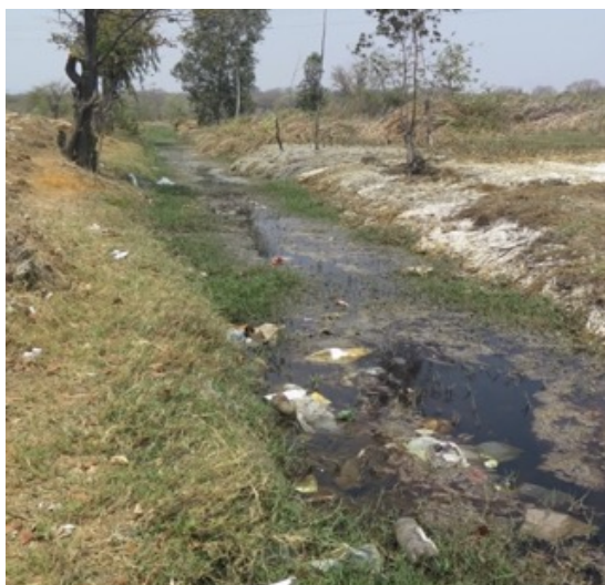
Suppl.-Figure 26 Effluent channel close to AMD point source on top of abandoned underground mine at S062/EFFCHI02 at 18°20'6.45"S, 26°28'13.37"E. Picture taken on 23.09.2019
