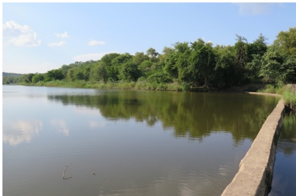
Suppl.-Figure 17 Deka River at S002/UPSDEK02 showing dam upstream of confluence with Sikabala channel. Picture oriented North, taken on 02.02.2019 at 18.2848 S, 26°29'51.03"E
