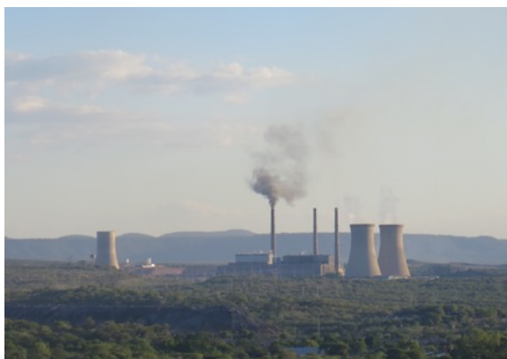
Suppl.-Figure 44 Thermal power plant in Hwange with mine waste heaps in front. Picture taken on 30.04.2019 from 18°20'39.93"S, 26°30'12.07"E looking South West
