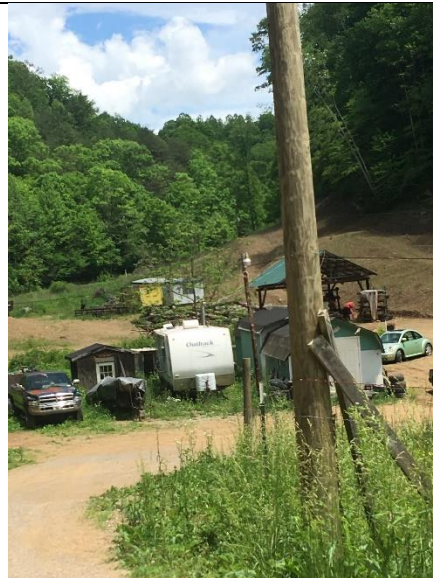
DF#3 focus area of severe erosion
