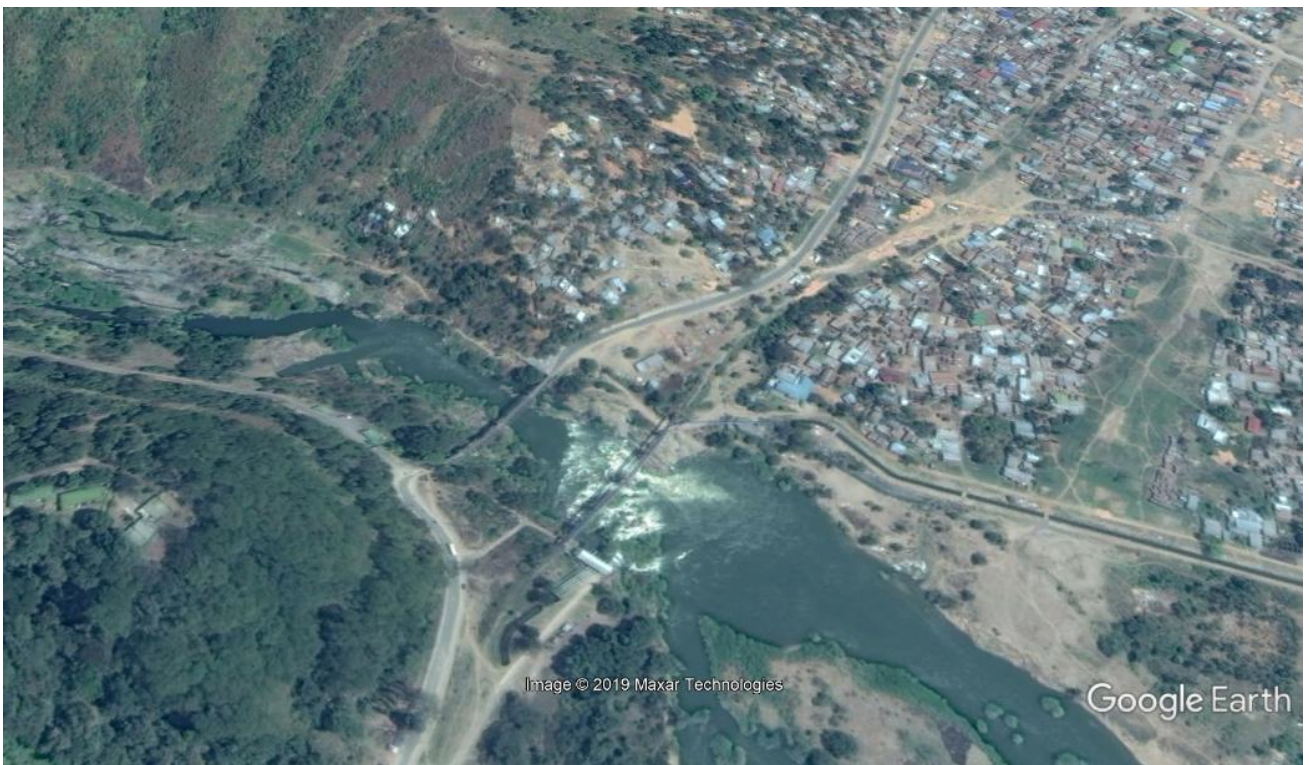
Figure 77: The Great Ruaha river near Kidatu, showing road and rail bridges (-7.663, 36.979).
