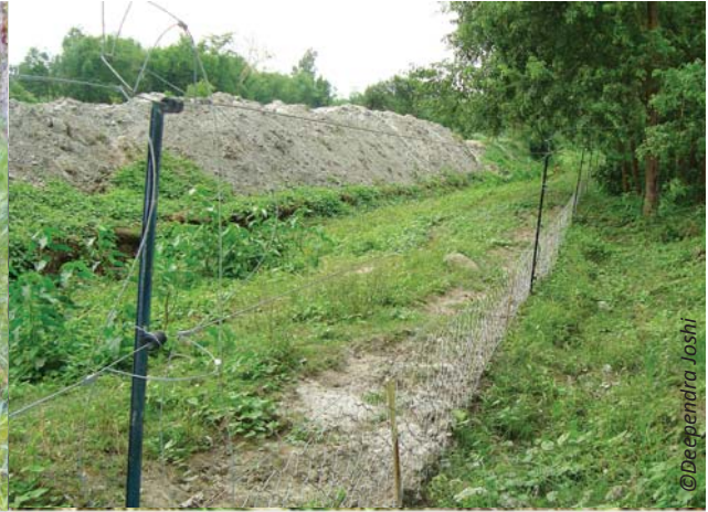
Solar fencing constructed to reduce human-wildlife conflict
