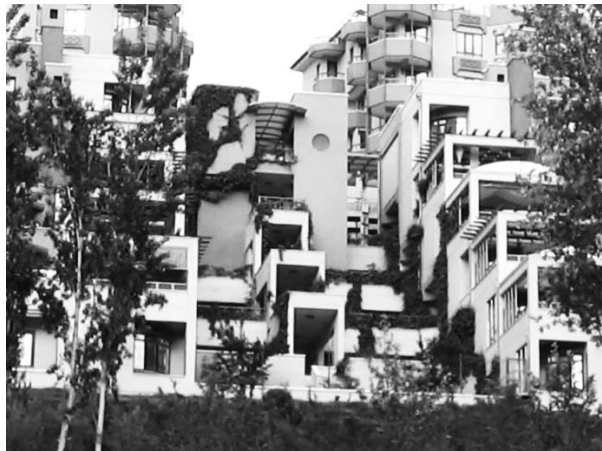
Figure 7: Green roof and green wall as stepping stone between the patches (Original).
