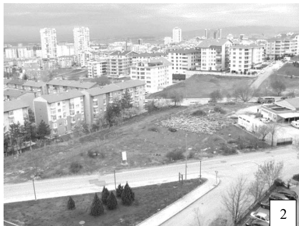
Figure 5: The construction process of site, elimination of natural vegetation (Ankara-Original).
