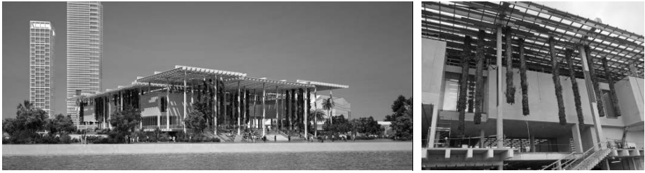
Figure 10. A:Application example of hanging system, Miami Art Museum (URL-9), B: Hanging system combination with façade (URL-10)
