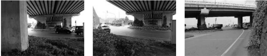
Figure 12. Planting and posters exist where the viaducts' columns join the road
