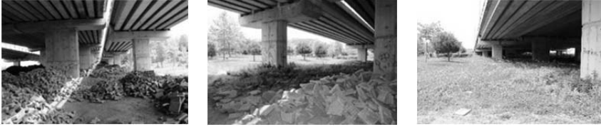
Figure 11. Not organized empty space under viaduct and picnic area
