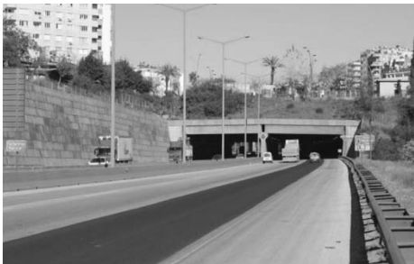
Figure 2: TAG highway retaining wall
