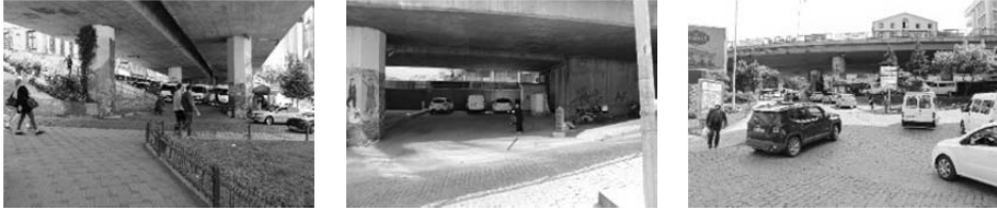
Figure 14. Share taxi and parking area under Tanjant Bridge
