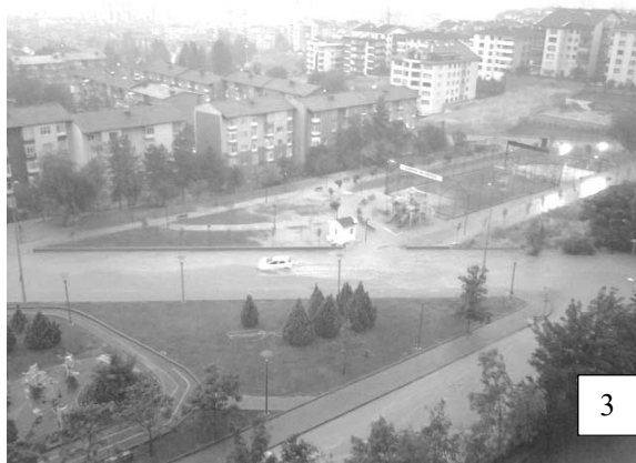
Figure 6: Result/ flooding area; the construction process of site, elimination of natural vegetation in 2015 (Ankara-Original).
