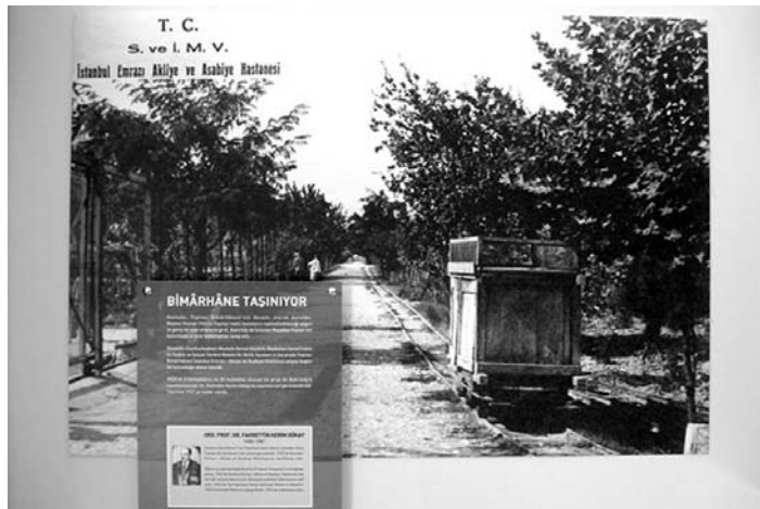
Figure 14: Old picture of hospital road (Anonymous, 2015a).
