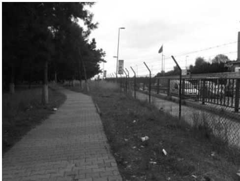
Figure 3: Wire fence and concrete pavement lock (Original, 2014).
