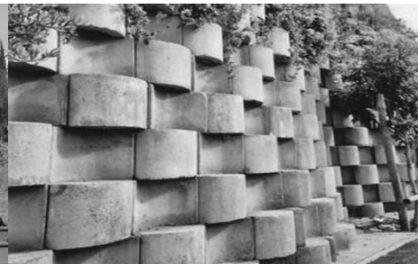
Figure 3: Alternative retaining wall
