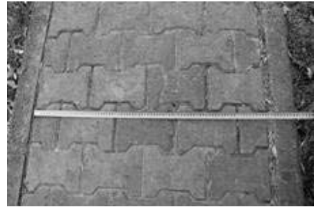
Figure 7: 80 cm wide walkway (Original 2016).
