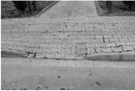
Figure 10: Disabled ramp allowing the entrance to the Park (Original 2016).
