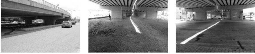
Figure 7. Reşadiye-Moloz Overpass space
