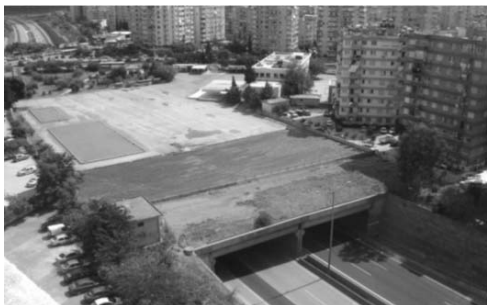
Figure 4: TAG highway model cut -cover tunnel
