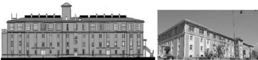
Figure 6. Tekel Tobacco Warehouse Restoration (Western View 1/50) (TKB & ÇEKÜL, 2013)
