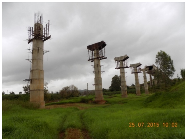
Fig. 2 Construction of Water canal
