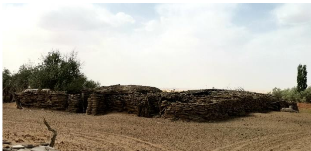
Fig. 10 Stock barns made of Haloxylon ammodendron (C. A. Mey.) Bunge (Taken by Liu in Ejina)
