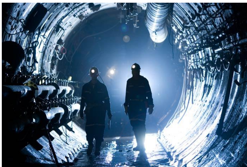
Figure 21: Underground development at Cigar Lake. Cameco has developed underground tunnels or drifts, reinforced by concrete to prevent water inflow and provide stable ground for mining.
