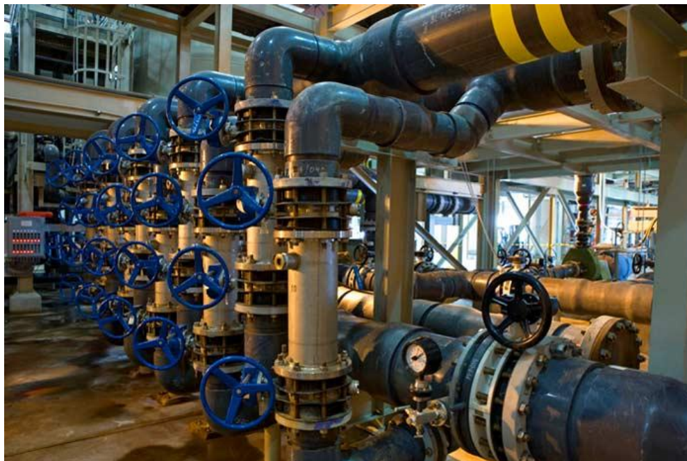
Figure 15: Closed loop recirculation system is used to dissolve and recover uranium.
