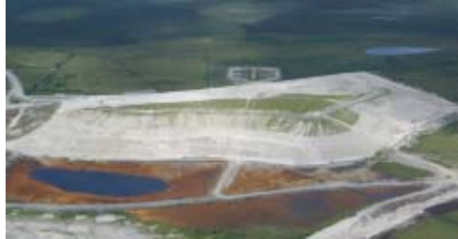
► Waste rock pile at Selbaie Mine with acid collection pond in the foreground. The area of release from ditches is in the top right corner.
