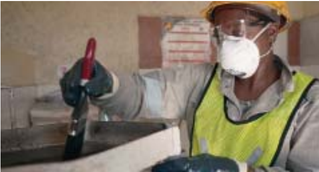
► Maduka Construction employee working on stonedust barrier
