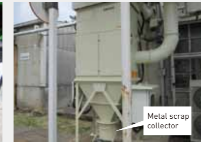
Fig. 2. Metal scrap deposited in dust collectors
