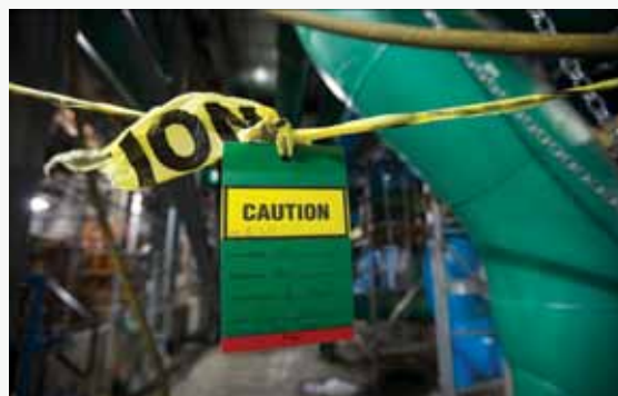
A caution tag and yellow caution tape are used to safely cordon off an area where maintenance is being performed.
