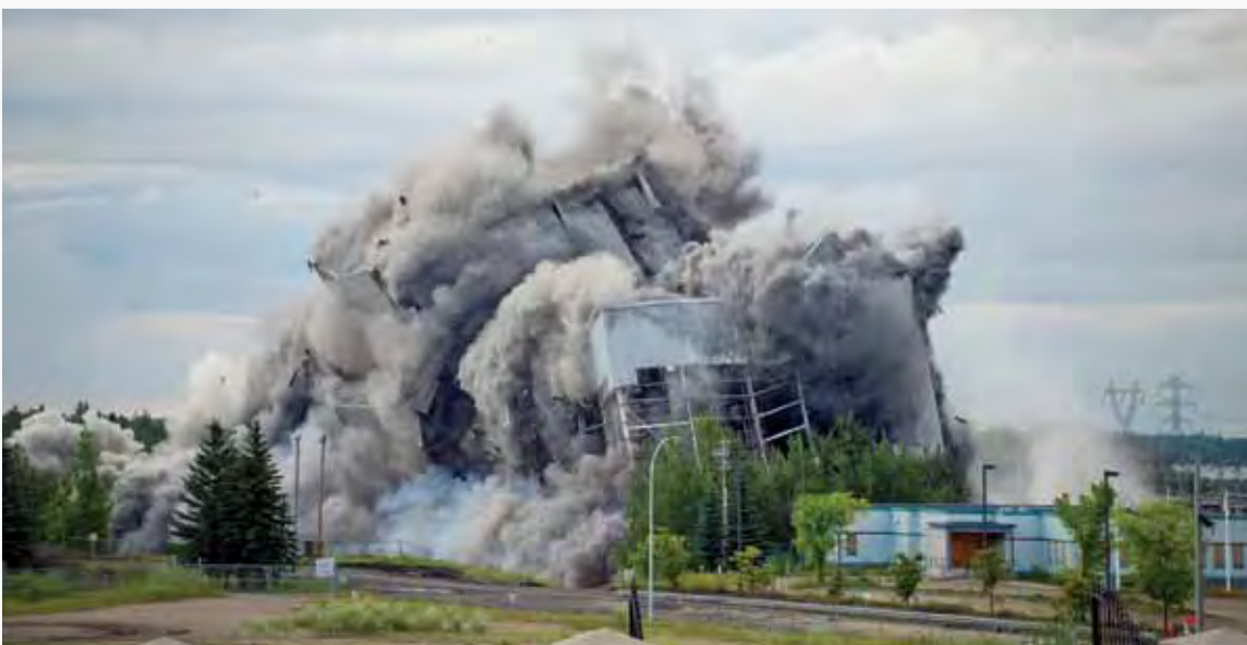
The Wabamun coal-fired power plant was safely imploded on August 11, 2011.
