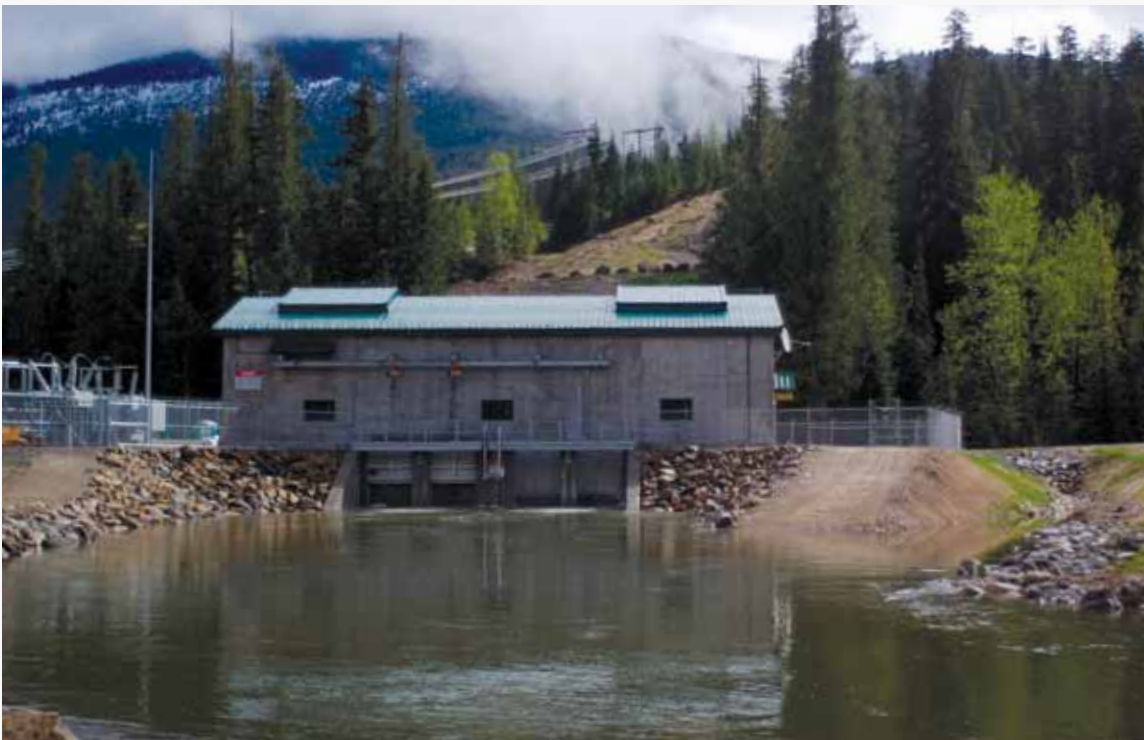
Bone Creek, a 19 MW run-of-river hydro facility, located near Blue River, British Columbia.
