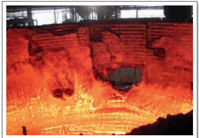
Figure 7. Intact preassembled slag door after 346 heats.
