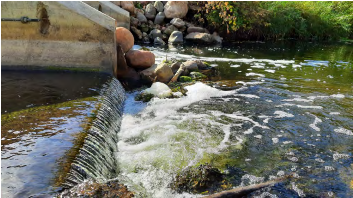
Figure 4 Culvert on Rice Creek
