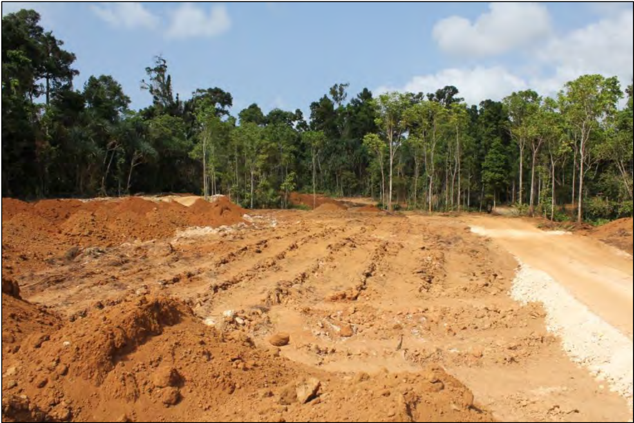
Figure 4: Photograph showing rip lines and paddock-dumped soil mounds
