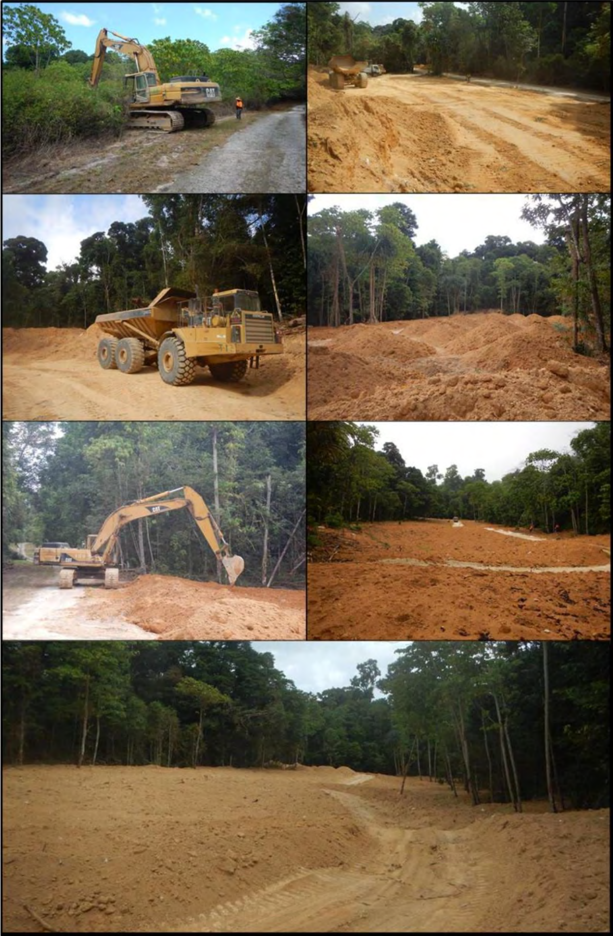
Figure 3: Earthworks at Blowholes Field 107
