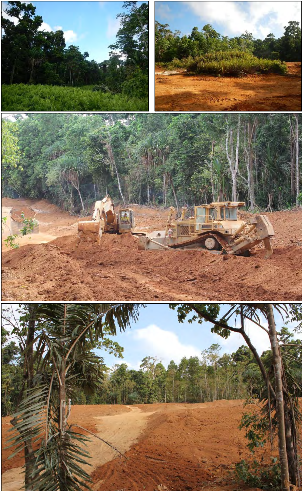
Figure 3: Earthworks process at Field 23 North- before, during and after
