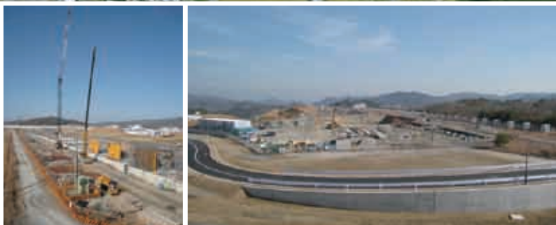
XFEL facility under construction
