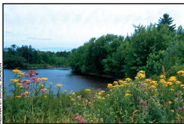
HIGHWAY 61 BRIDGE, SCANLON
