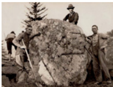
Fig. 4 The largest boulder used for construction of the exotic rock garden, said to have been sourced from Scarborough. Walter Brockie is perched in the top middle of this photo. The other men are Ted Roe (left) and A. B. Tomes (right). This photo was taken around the time for the opening of the rock garden on 29 July 1939. Photo courtesy of Bob Brockie.
