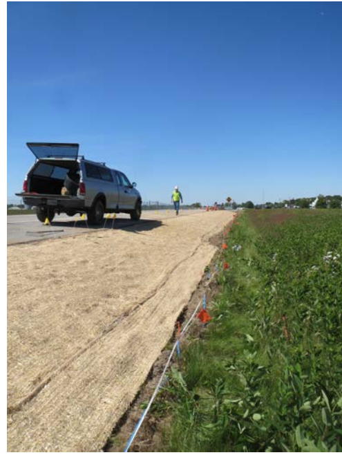
Figure 2. Photos of the Eastern Shore site (left facing south and right facing north). Existing vegetation was killed with glyphosate, the existing soil removed, and new soil added. Plots were seeded the same day that soil was added to the plots. A biodegradable straw blanket was installed immediately after seeding to prevent erosion and provide a better climate for seed germination.
