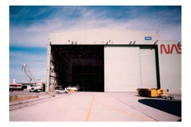
Chosen for safety and economy of operation, a CORYAVAC<sup>®</sup> system with eighteen cast iron "Classic" burners heats the NASA shuttle hangar at Edwards Air Force Base. Even in high bay buildings the fast warm up provides chill chasing warmth during cold nights and early mornings.
