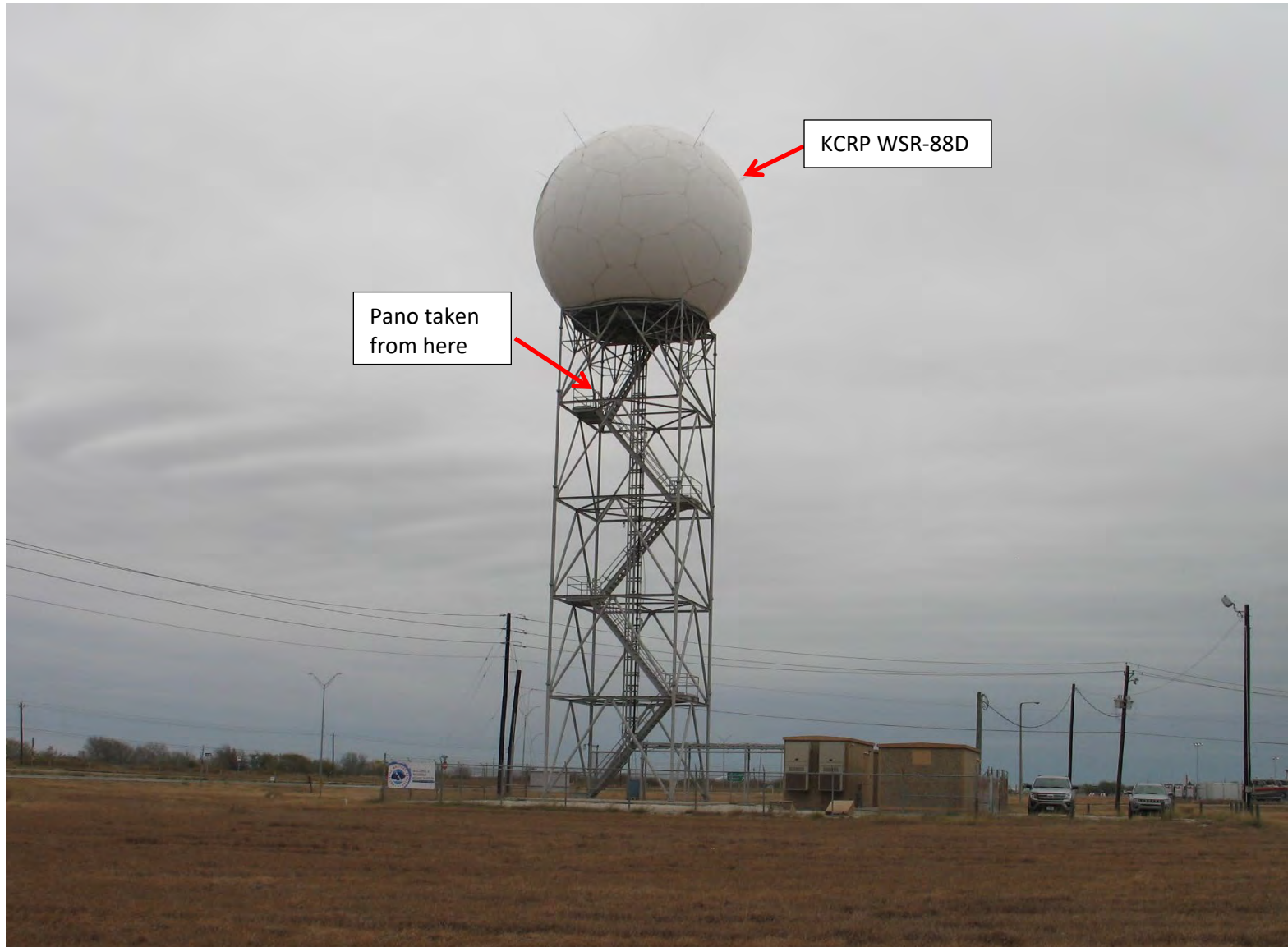
Photograph 1: KCRP WSR-88D serving Corpus Christi, area viewed from southwest.
