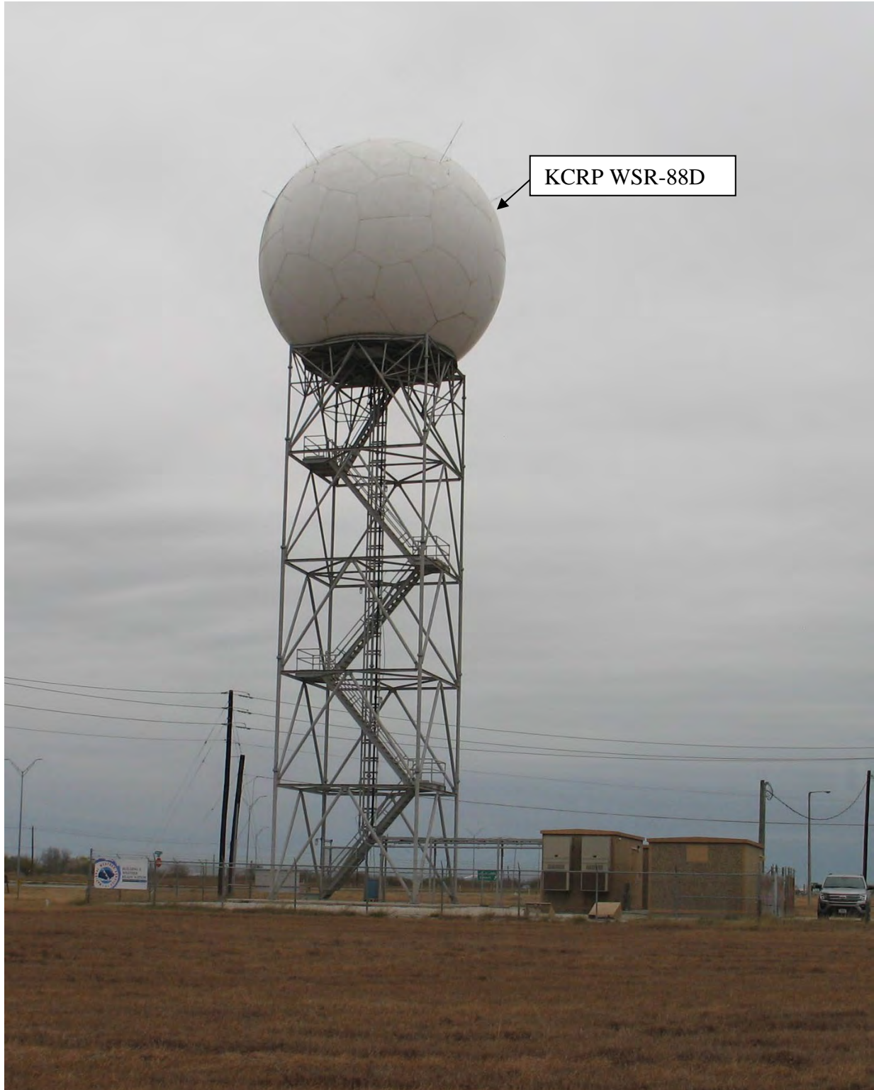
Figure 1: Photograph of KCRP WSR-88D serving Corpus Christi, TX, area
