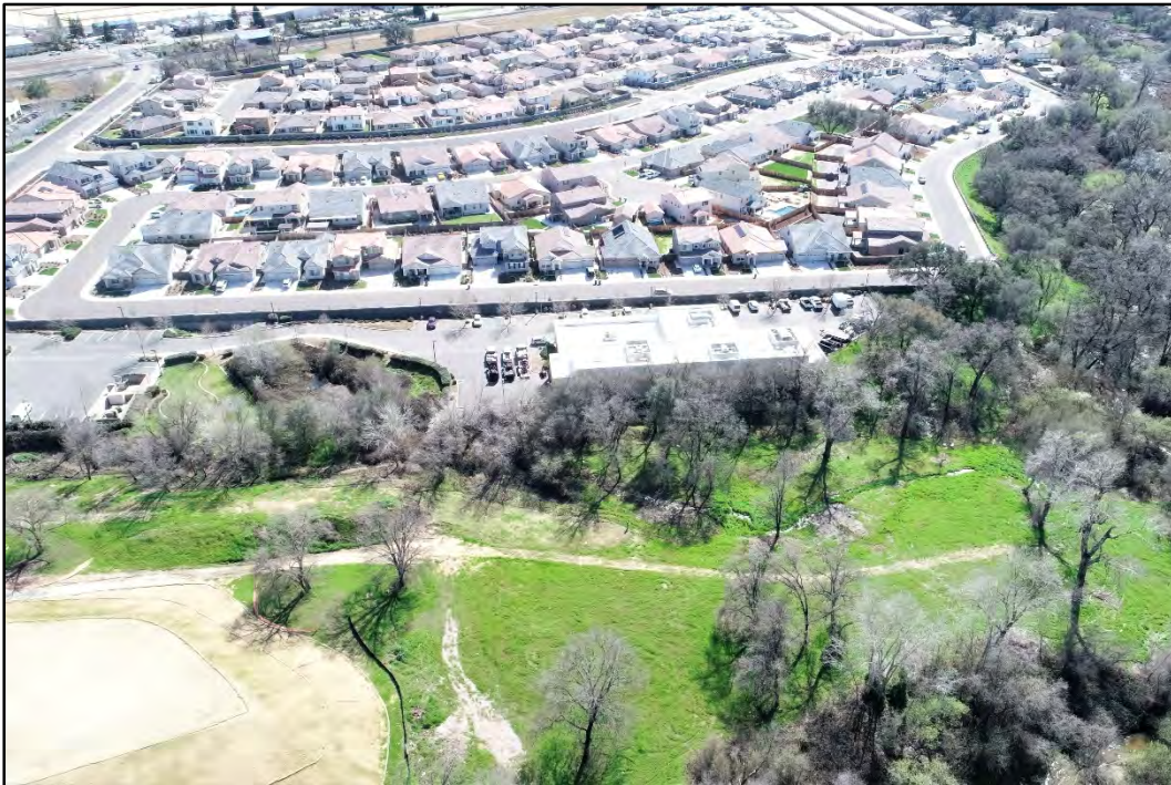
Looking south across property. Photo Date 6-4-19
