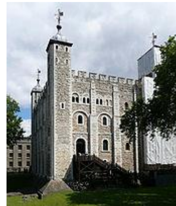
Figuur 95 Tower of London, originally begun by William the Conqueror to control London
