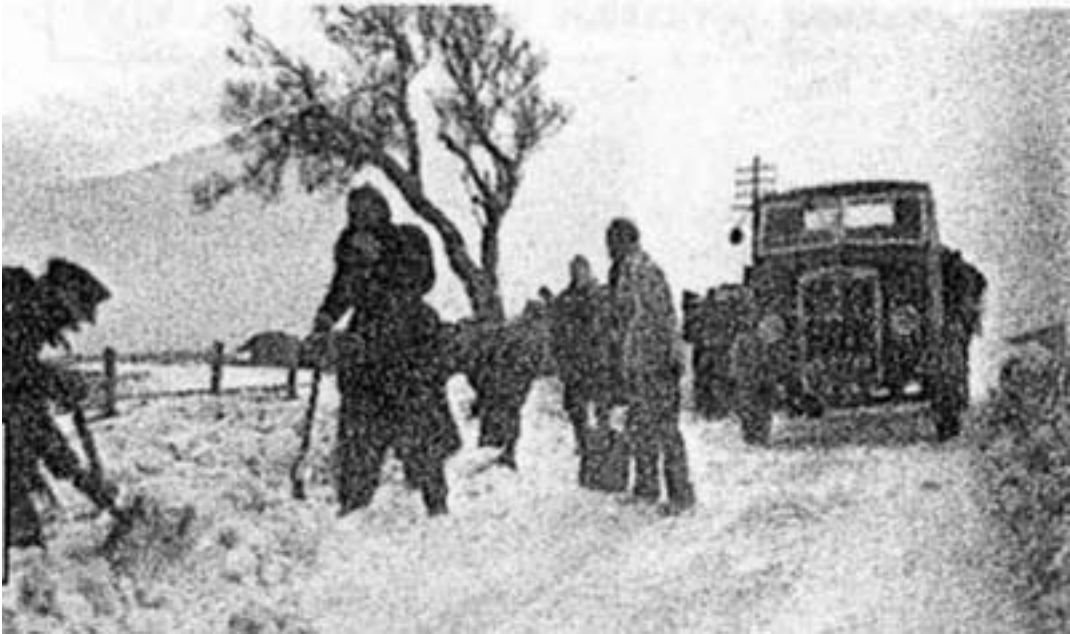
Clearing the road.
