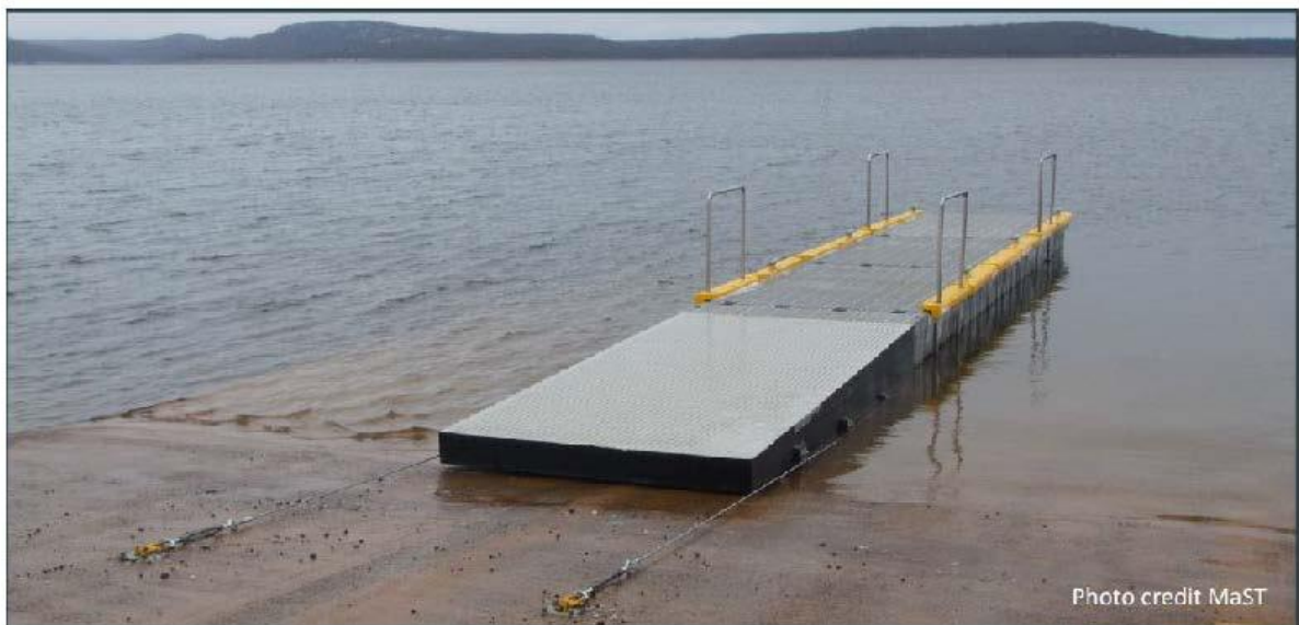
Brandum Bay (mid-cable position)
