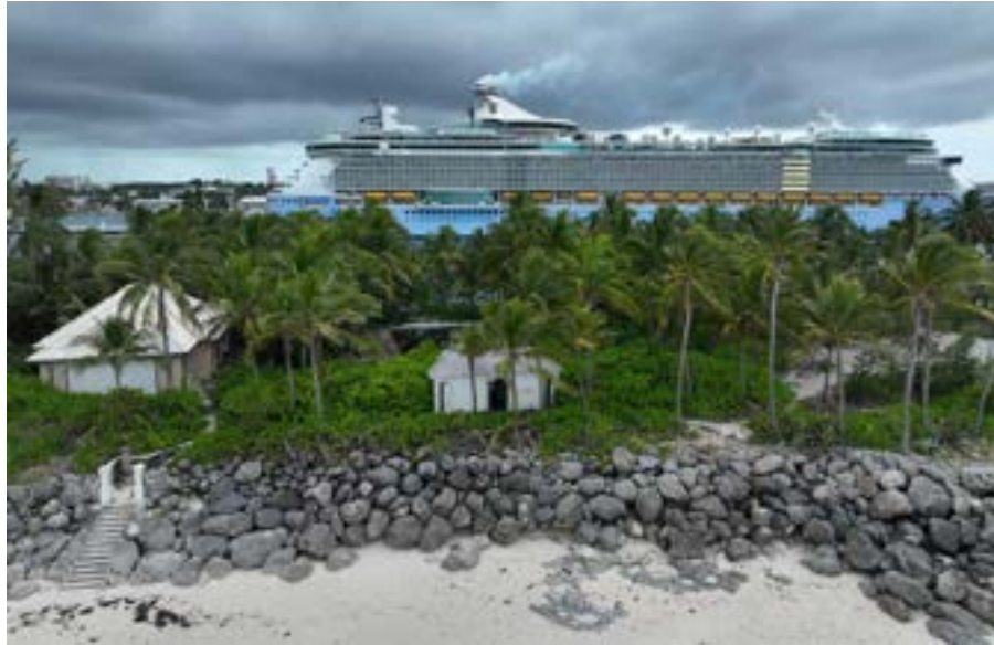
Photo 3-4: Rock revetment along Northern shoreline
