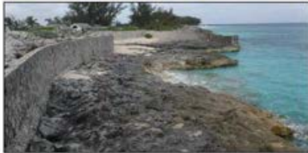
Figure 4b (left): Central shoreline, with high vertical ironshore, and existing seawall along eastern half of central shoreline.
