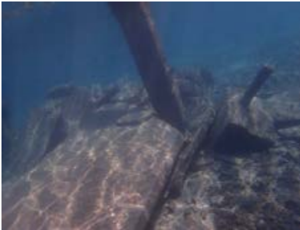
Photo 21: Collapsed dock on the southern side of the property
