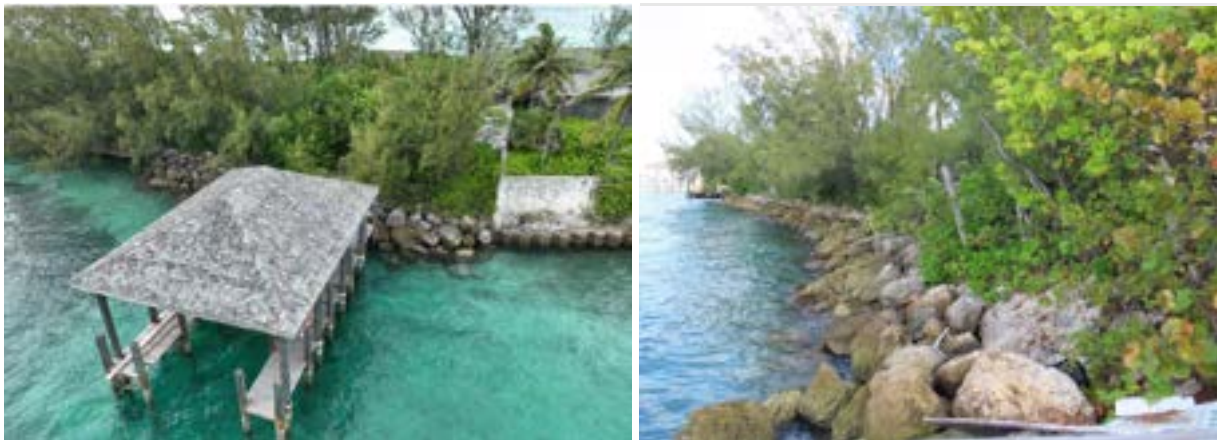
Photo 3-5: Rock revetment along Southern shoreline
