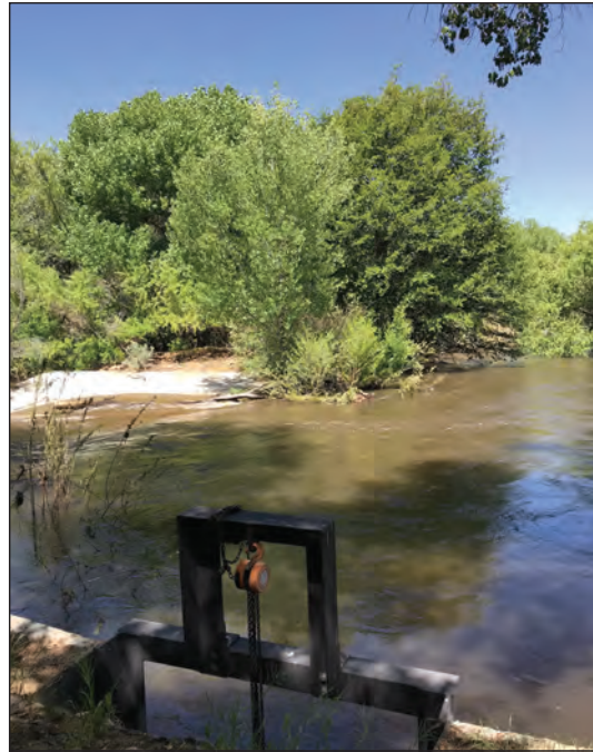
PHOTOGRAPH 5: An existing diversion structure (Nicoll Ditch) located on the Kern River.
