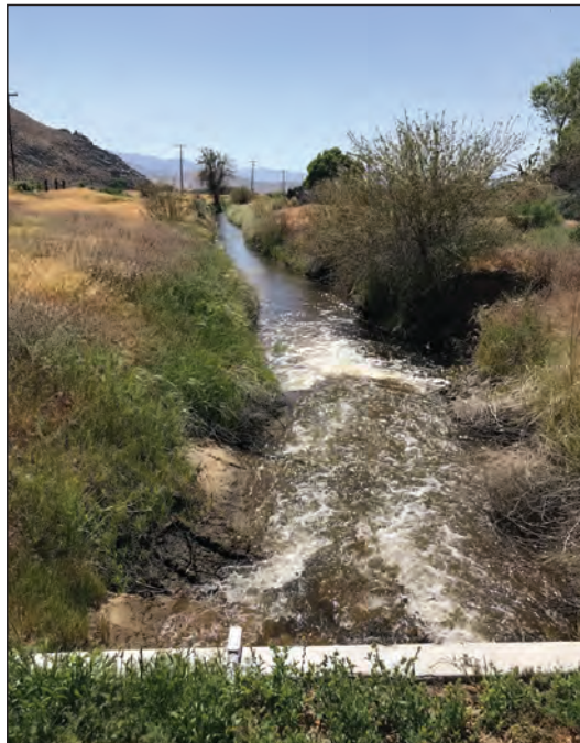
PHOTOGRAPH 6: Mack Ditch downstream of Nicoll Ditch connection.
