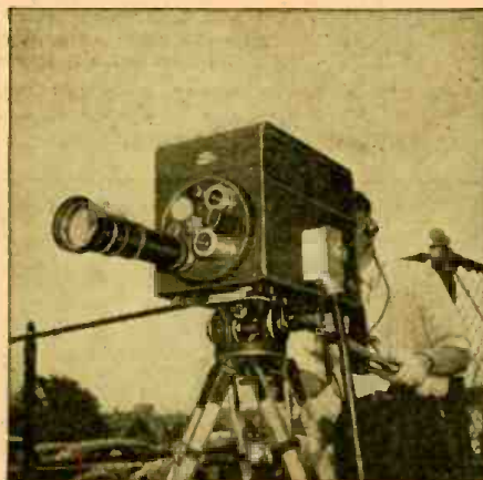
Orthicon camera for small telecasters—can be used both for outside pickup and studio work.
