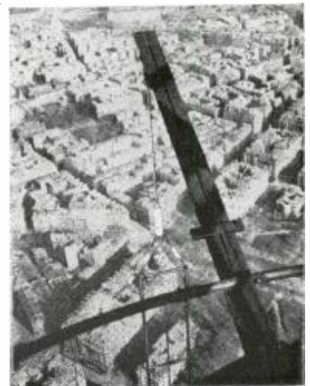
Ladder is insulated to avoid r.f. absorption.
