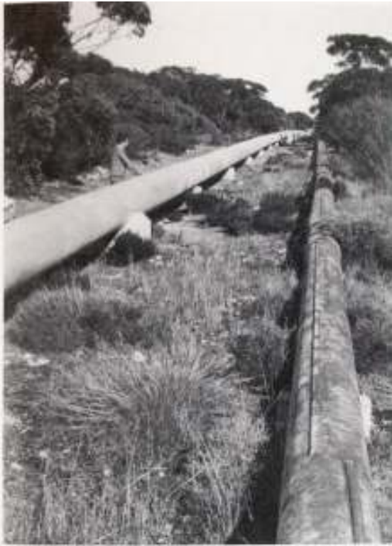
Fig. 7. The provision of water for stock and for other purposes was another boost to the settlement and development of the Peninsula. But the waters of the Tod Reservoir proved too corrosive for the first pipeline constructed, and it has been gradually replaced and enlarged. The two, the old and the new, are seen side by side here between Minnipa and Ceduna. (E and W S Department).
