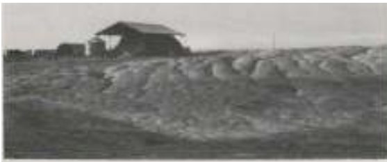
Fig. 29. Dumonte Reservoir north of Wudinna, showing the channels of the naturally exposed rock, continuing in the natural subsurface.
