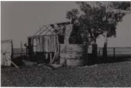
Fig. 11. Ruins of abandoned homestead, south of Minnipa. Note the materials used—corrugated iron and local split timbers, and of course the rain tank.
