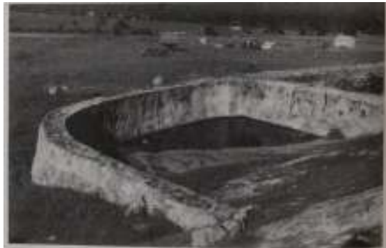
Fig. 10. This small storage was built at the base of Kolbatta Hill. Though it leaks it nevertheless still holds water for many weeks and is therefore useful in this dry country.
