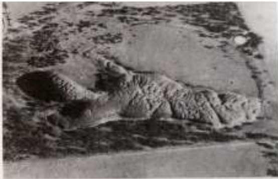
Fig. 9. Many of the granite outcrops of northwestern Eyre Peninsula provide excellent catchments, for the massive rock of which they are made is essentially impermeable. The State Government utilised many of them for water conservation and supply. Pildappa Hill is a typical example of such a local but important conservation scheme. Low walls have been built around the lower margins of the hill. Run off is thus diverted into channels carefully levelled so that the water runs under gravity into large tanks or storages.
