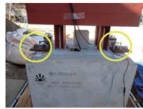
Yellow circle: microtremor sensor (installed at two locations on top end of bridge pier)
