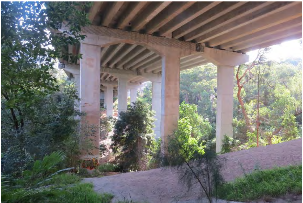
Figure 29 M2 underpass at Terrys Creek
