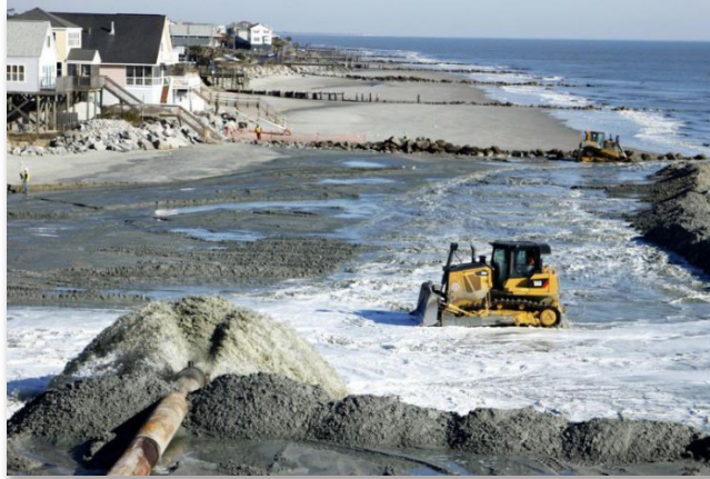
Figure 12 Folly Beach Pipeline Placement Operations 2019. Photo by: Sara Corbett
