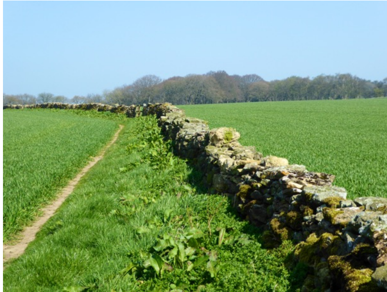
Figure 21. The wall constructed by the Duke of Leeds in 1735 across East Ayton Moor.
