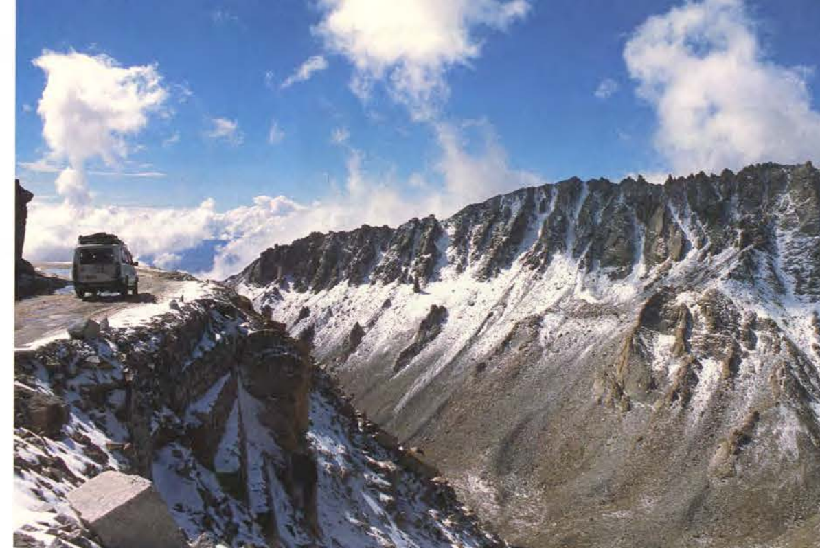
Photo 3: Opened in 1973, Khardung La (Pass) is claimed to be the highest motorable road in the world
