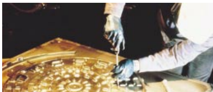
Inspecting a manhole.
