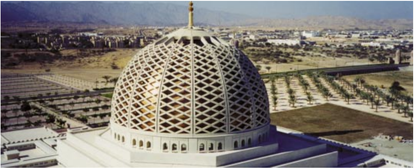
The Great Mosque of Oman, built using cement slabs reinforced with Cemfil® glass threads.
