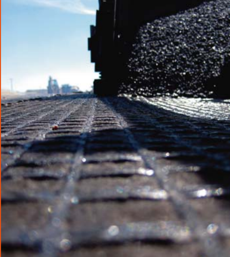
GlasGrid® paving reinforcement from Saint-Gobain Adfors protects asphalt roads, airport runways and bridges from cracks.
