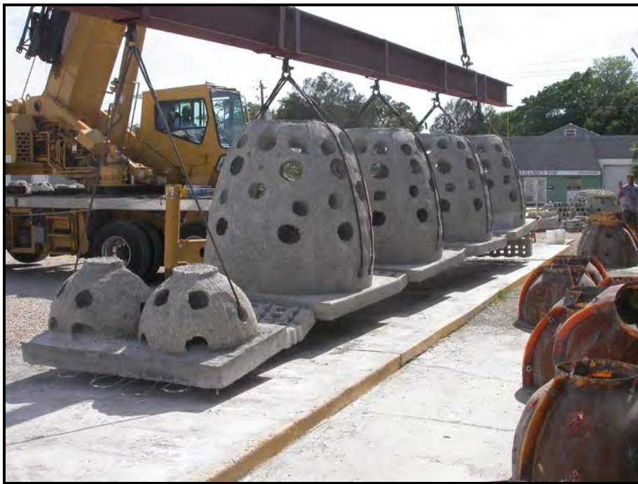
Figure 9 - Reef Balls molded to concrete blocks and connected into an articulated unit.
