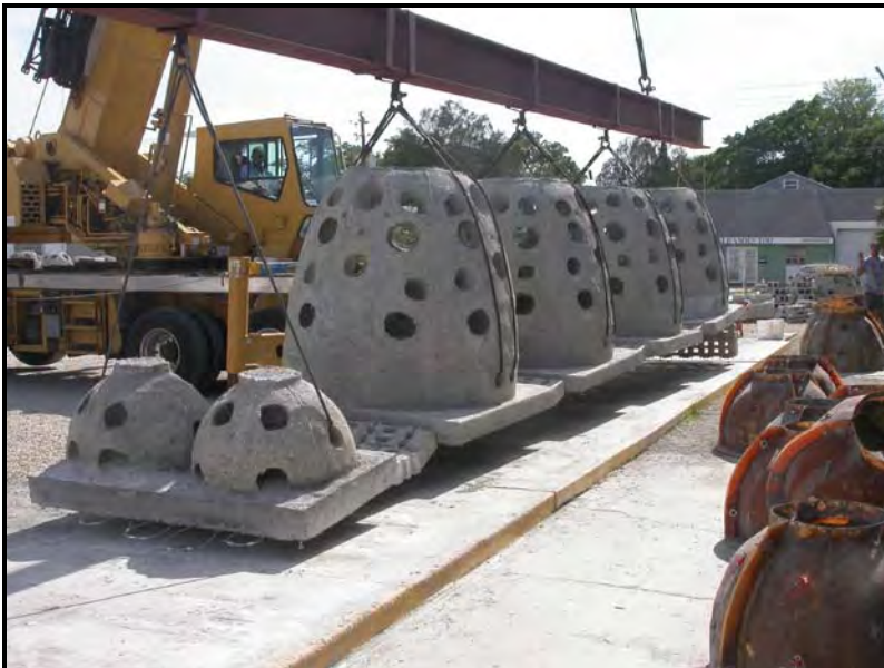
Figure 2: Reef Balls molded to concrete blocks and connected into an articulated unit.
