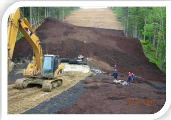
Technical reclamation of the right-of-way
