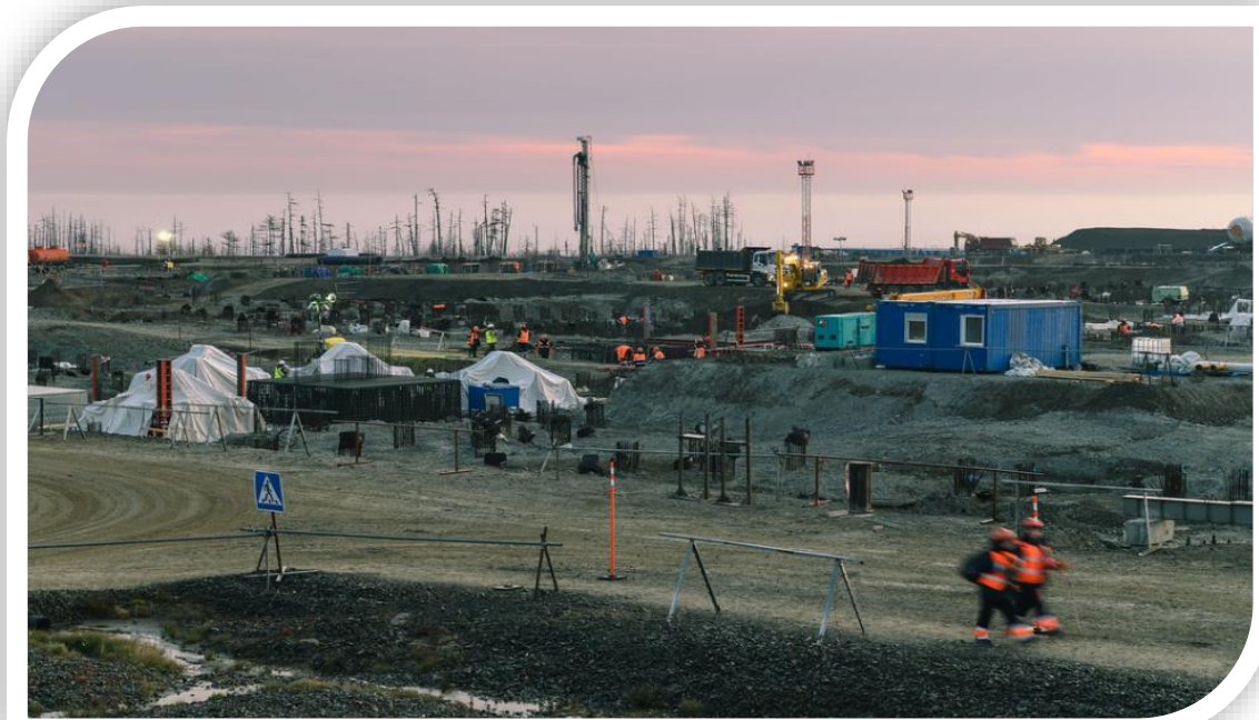
Construction works of the OPF-C project
