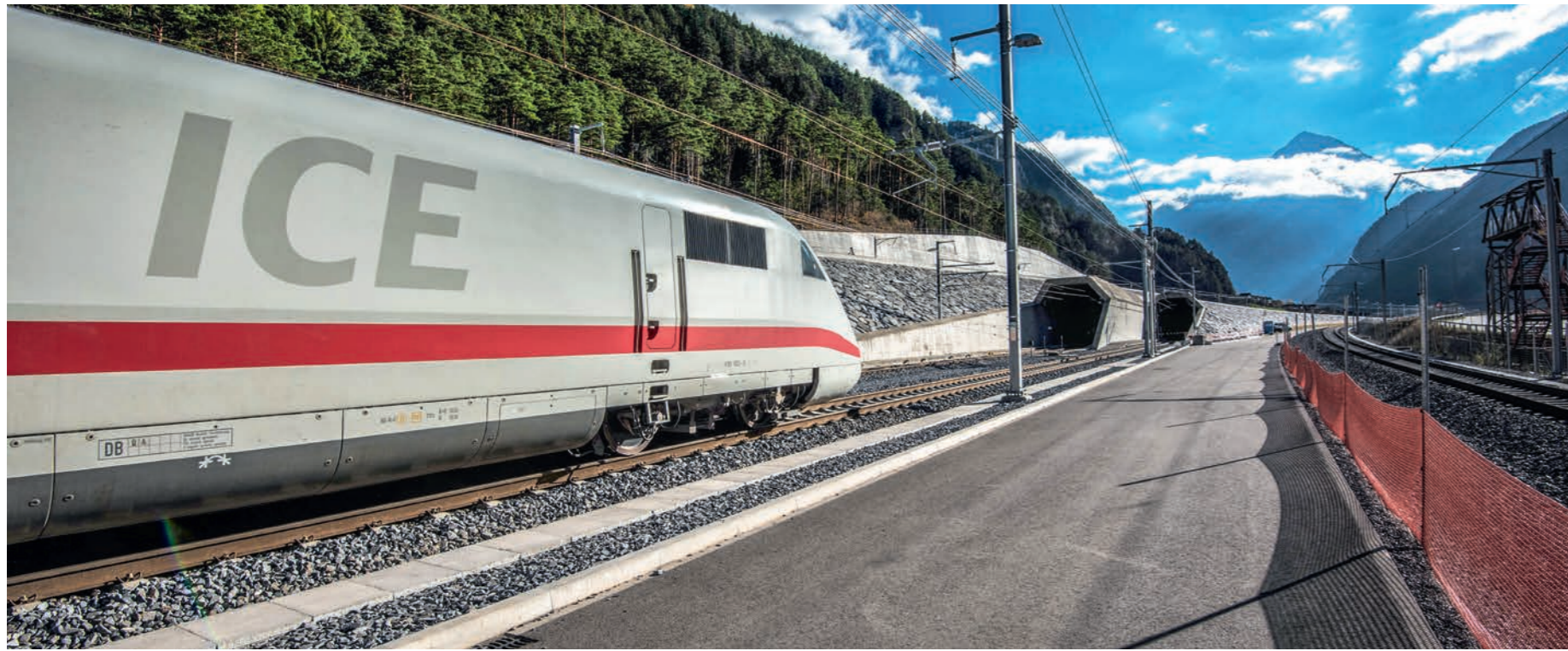
Passenger trains can pass through the tunnel at a speed of up to 250 km/h. They are to run every half hour, and shorten the travel time between Zürich and Lugano by 45 minutes
