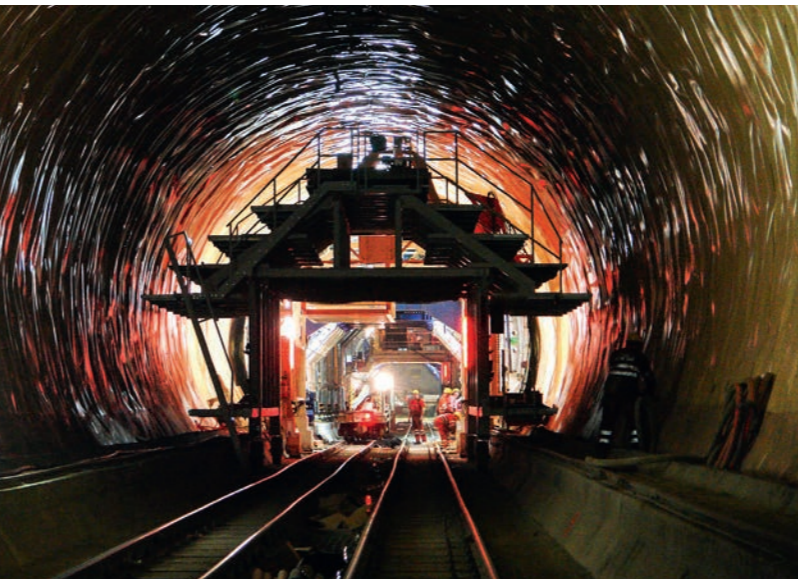
Photo: © Alptransit Gotthard AG
