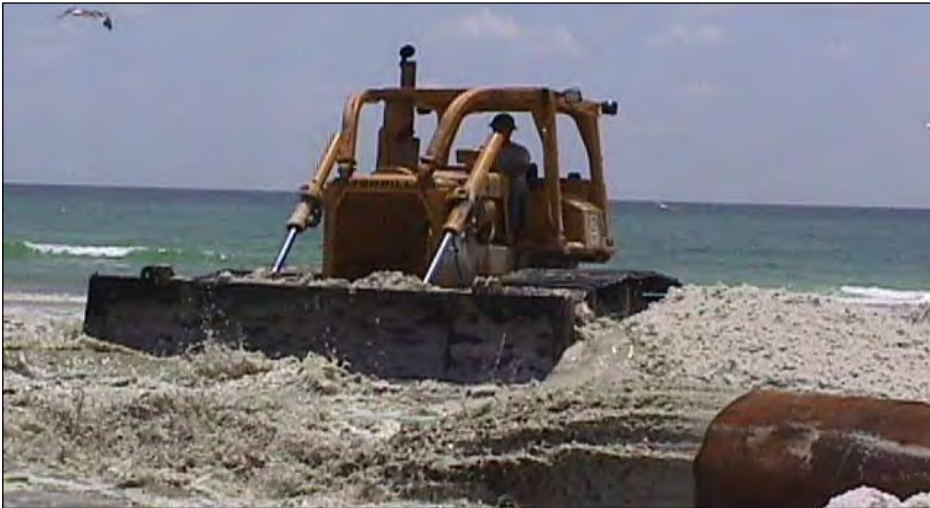
Pipeline Dredge Discharge
