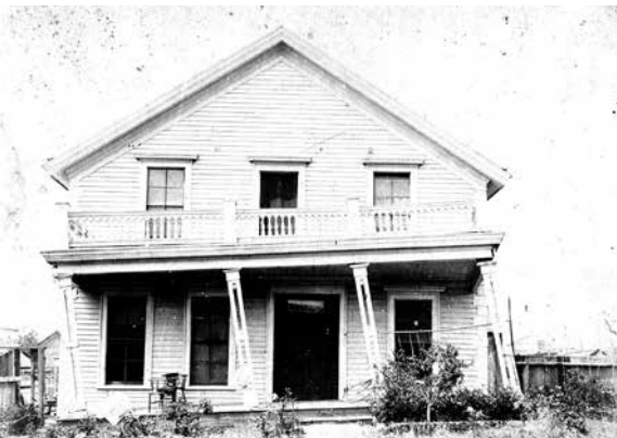
1906 San Francisco Earthquake leaves a somewhat twisted historic Zaballa House
