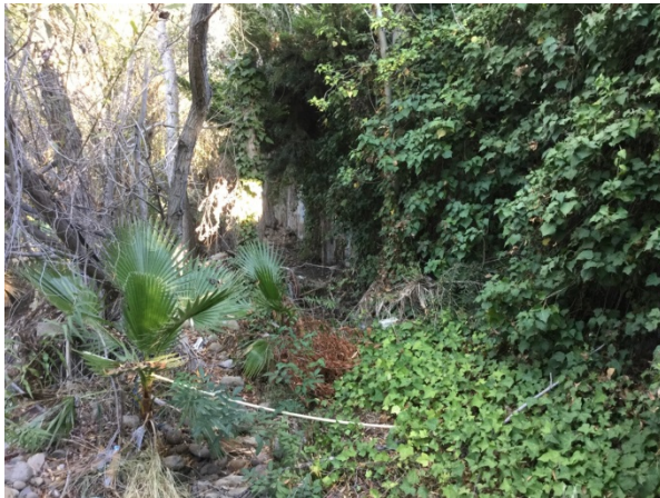
Reach 2 viewing north-east at the channel left bank, concrete wall (viewing downstream) and channel bottom.
