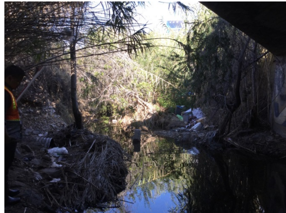
Downstream portion of Reach 2 viewing north-east at the vegetation and ponded water along the channel bottom.
