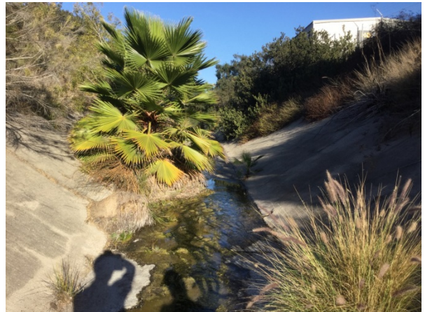
Downstream portion of Reach 3 viewing north-east at the concrete lined channel.
