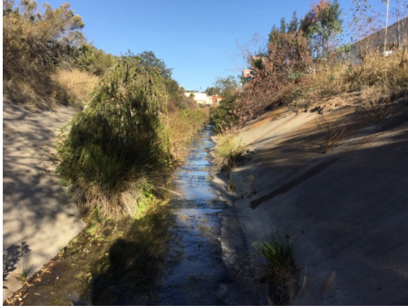
Reach 3 viewing north-east at the concrete lined channel.
