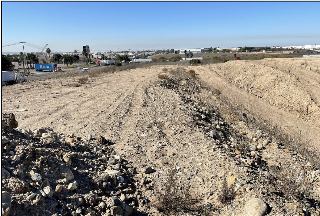
PHOTOGRAPH 2 View of Southern Stockpile Looking West (Photo Date November 15, 2021)
