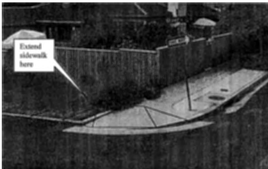
Photo 11b – NW corner
