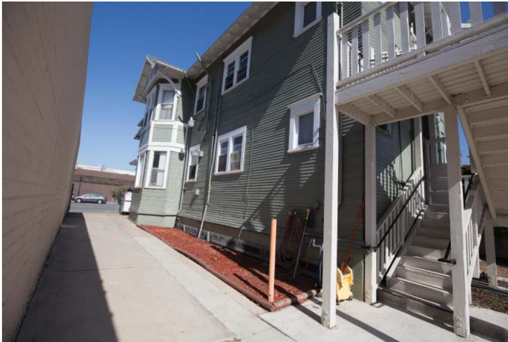
Figure 3-11: The Murray Apartments, view of the south façade.
