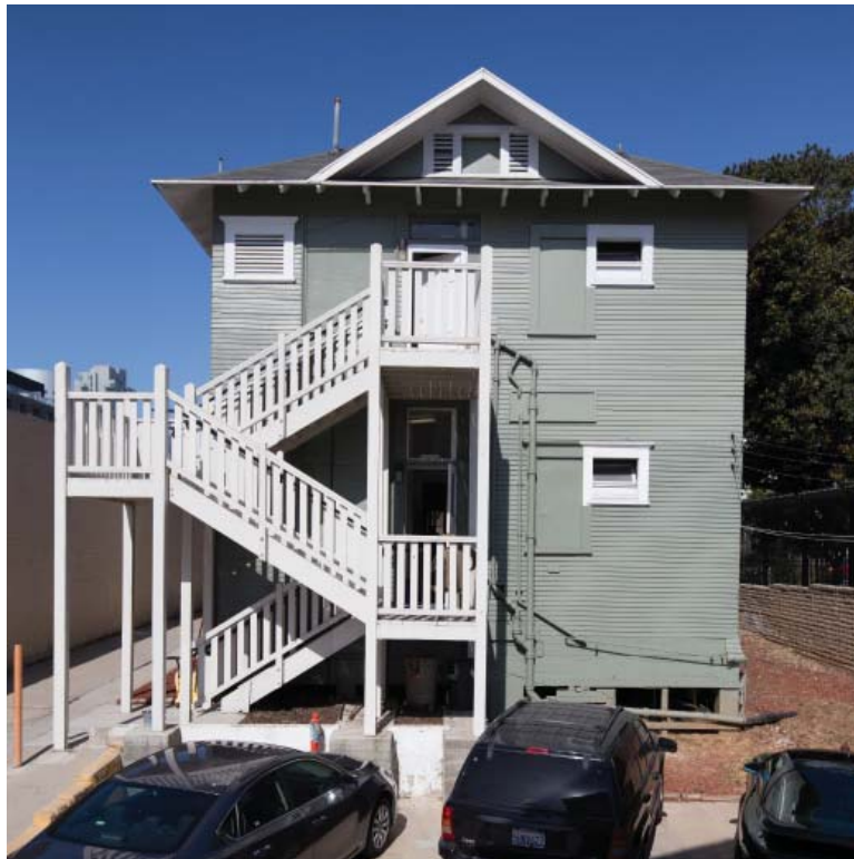
Figure 3-9: The Murray Apartments, view looking west at the east facade. Note the non-original exterior stairs and most of the fenestration has been in-filled.
