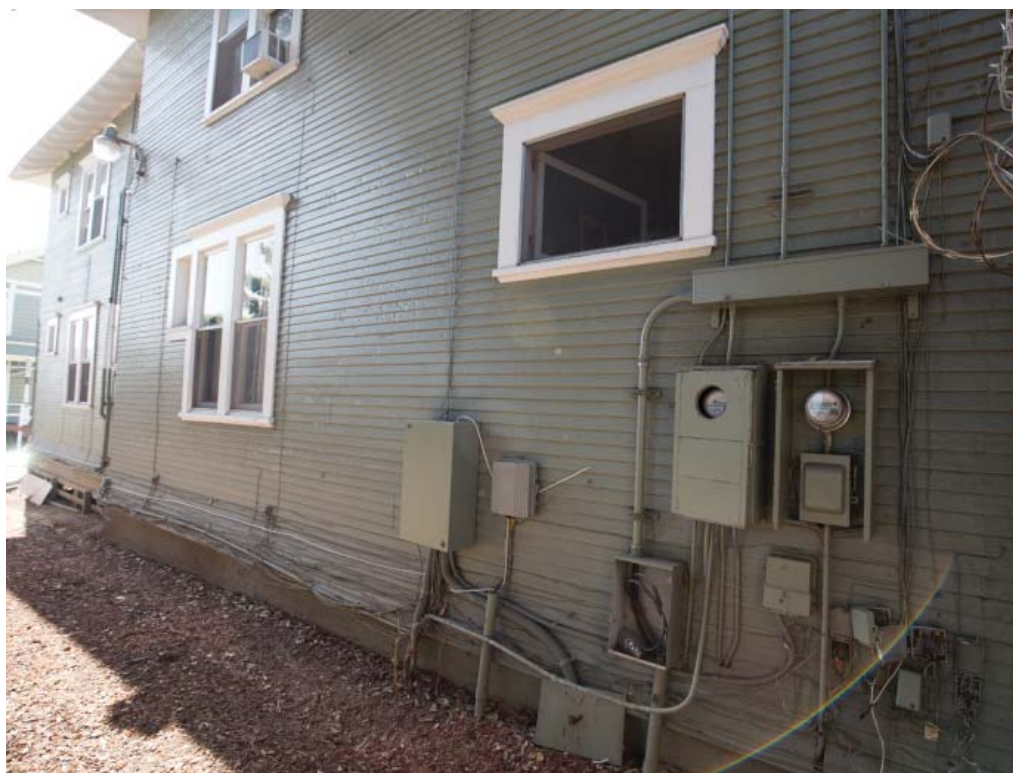
Figure 3-8: The Murray Apartments, view of portions of the north facade.
