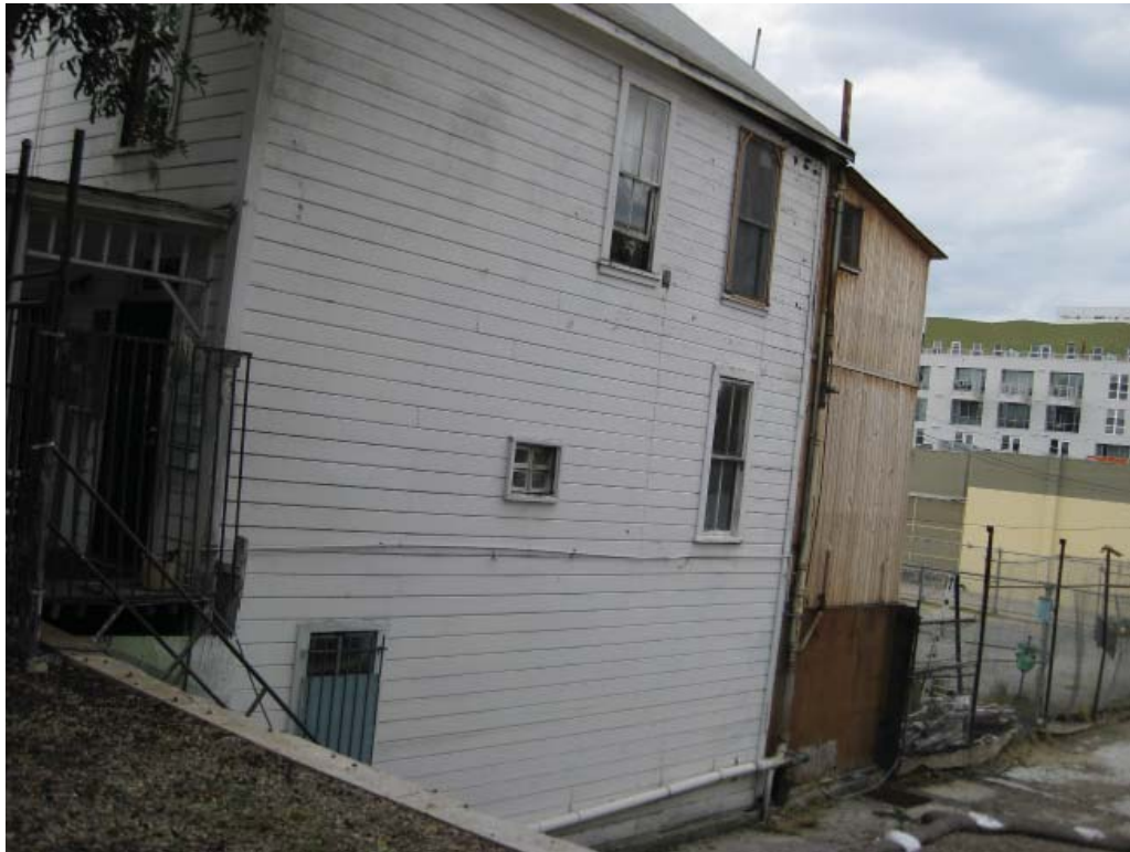
Figure 3-21: The Mattie Bearns House, view looking southeast at the west facade.
