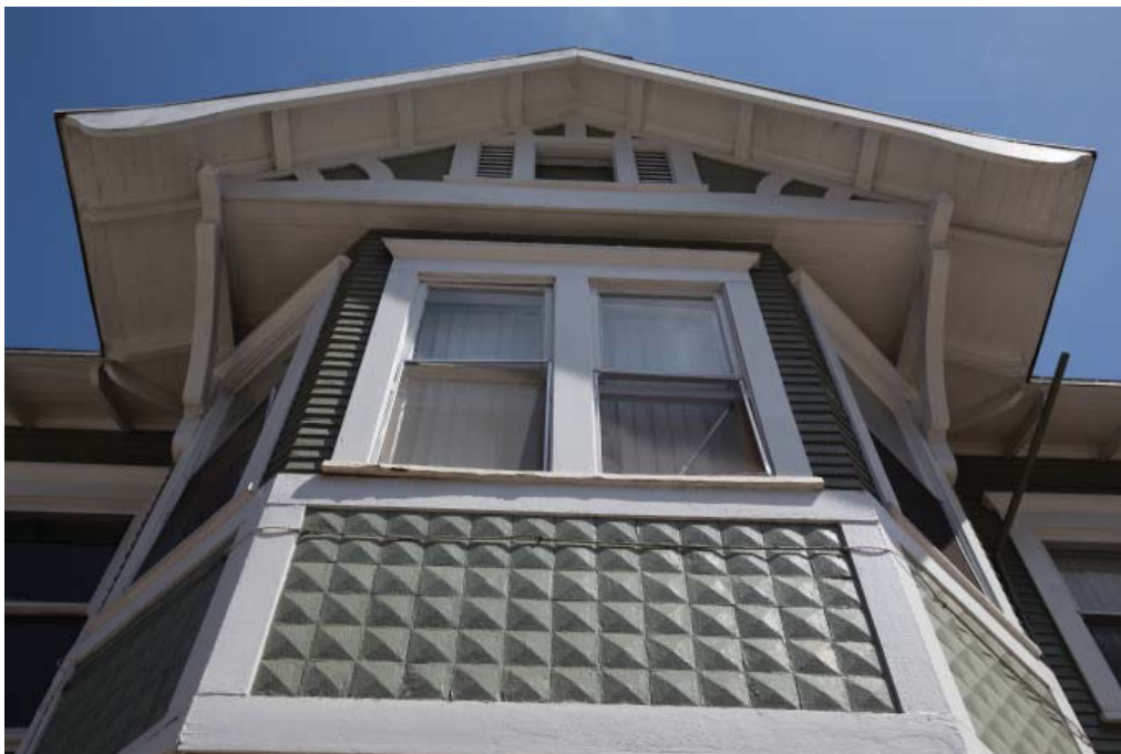
Figure 3-12: The Murray Apartments, detail at the south facade's second floor bay window, siding, and eaves.
