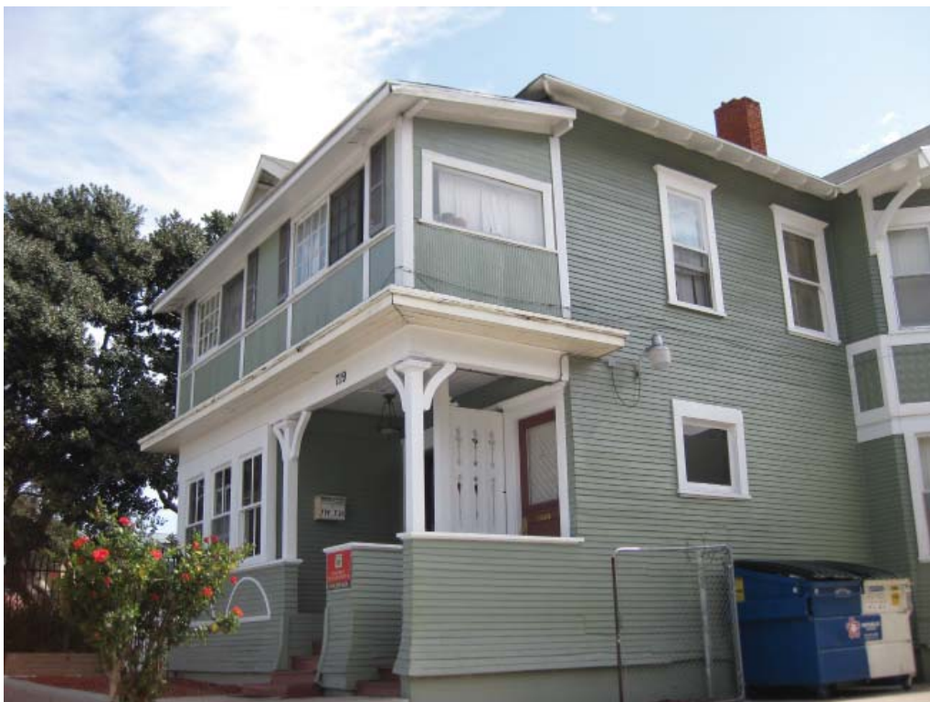
Figure 3-6: The Murray Apartments, view looking northeast at the porch. The second floor was extended on top of the original single-story porch.
