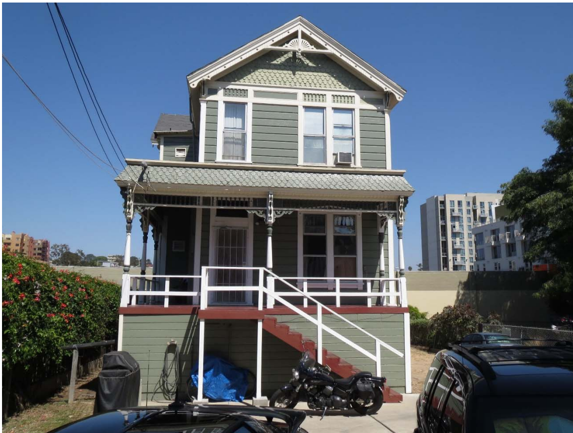
Figure 1: West facade of the Daggett Family Residence.
