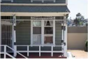
06_Porch Eave Detail
