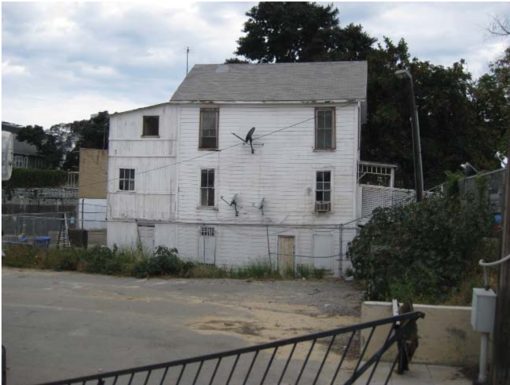
Figure 3-19: The Mattie Bearn House, view looking west at the east facade.
