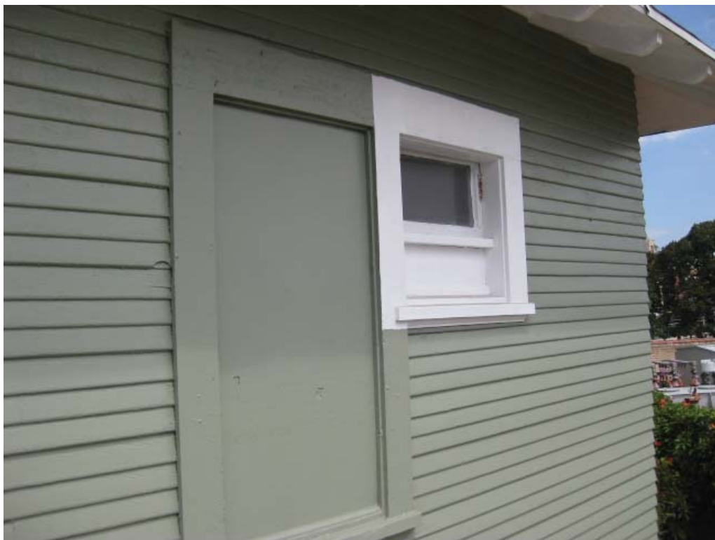
Figure 3-10: The Murray Apartments, detail of in-filled window at the east facade.
