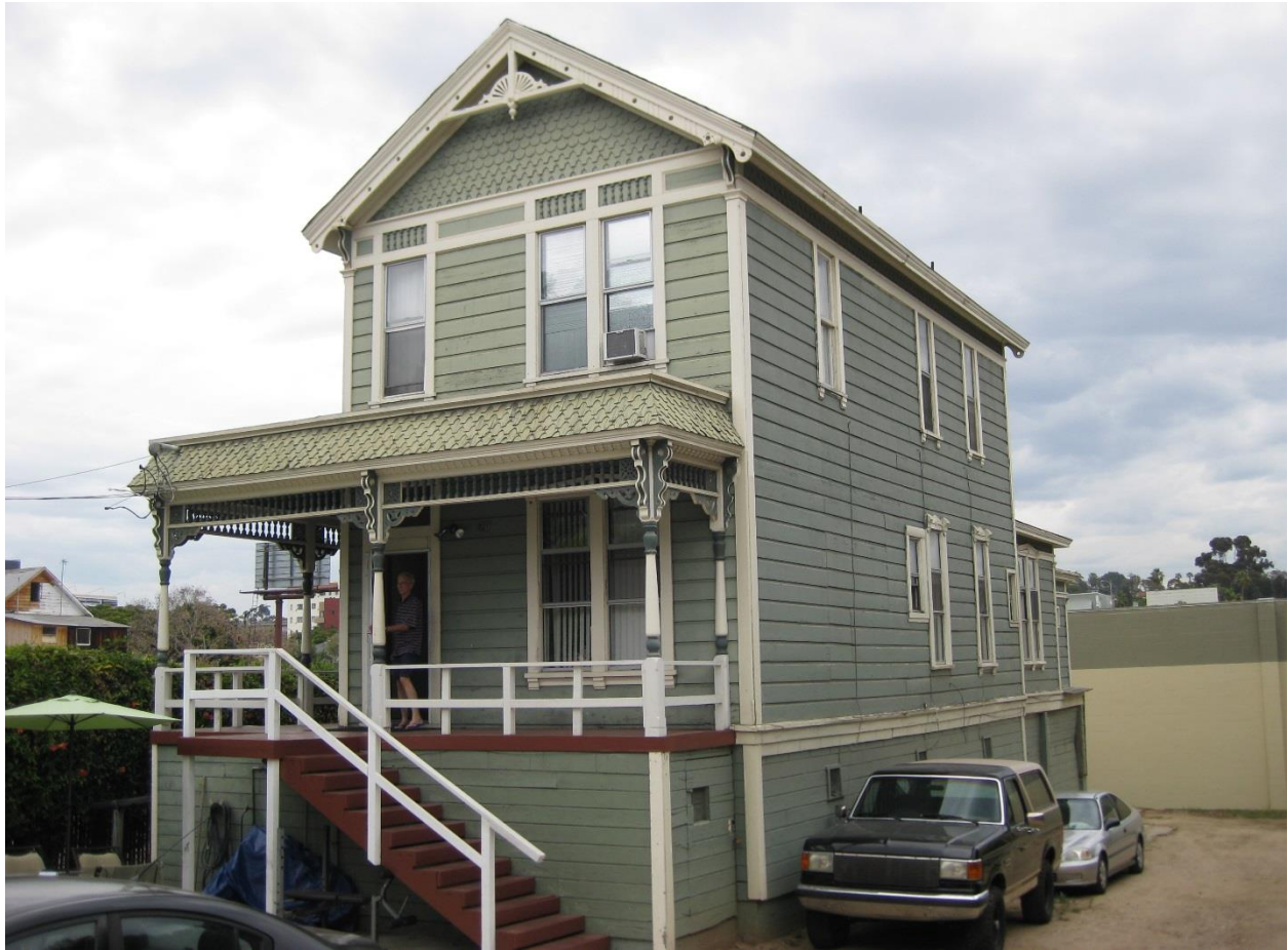
Figure 3-3: The Daggett Family Residence, looking northeast. Note the non-historic porch stairs which were added to accommodate the basement and garage which have been added below the original house. The entire house was lifted at least six-feet when it was moved to its present location at 721 14 th Street.
