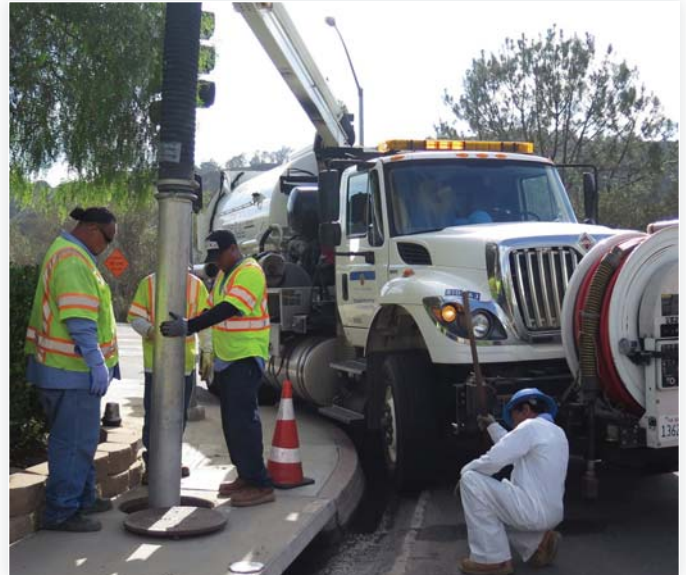
Street Pole Installation
