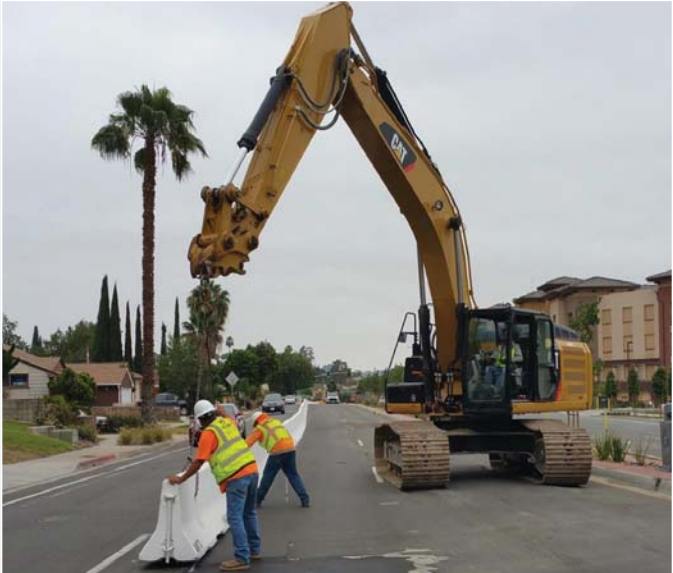
Public Works Department at Mission Gorge Road
