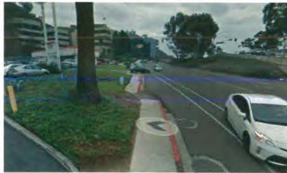
WEST DRIVEWAY-FACING WEST
