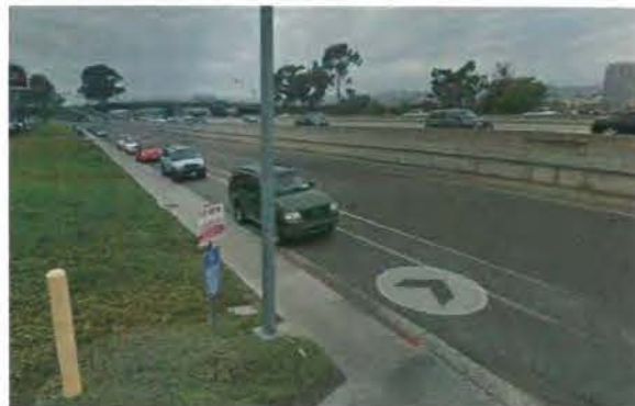
EAST DRIVEWAY-FACING WEST
