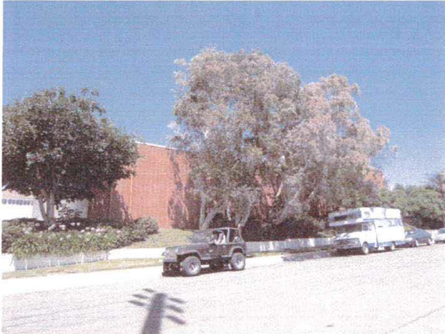
(1) View of the subject property looking north.
